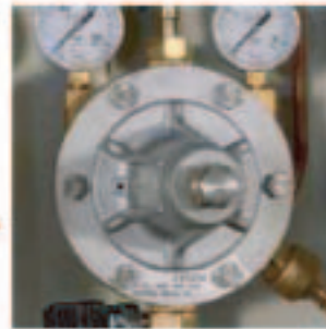
3rd Aux Source Cylinder Station 180 m 3 /h
