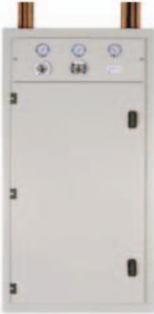
2nd stage Reducer Panel of 3 gases O_2 , Air, Vac (double reducers)
