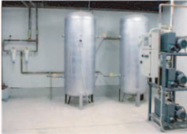
Medical Vacuum central station Vertical
